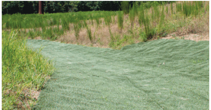
ShearForce10 channel installation
