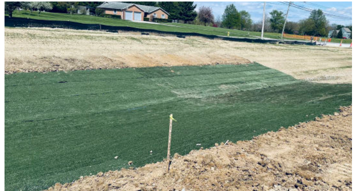
ShearForce10 Channel Installation
