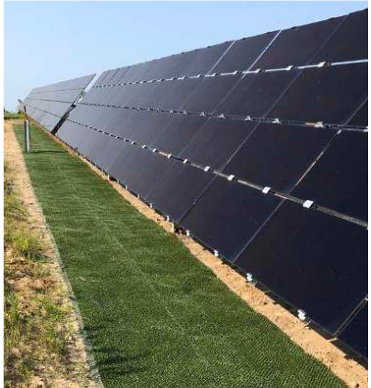
ShearForce10 dripline installation
