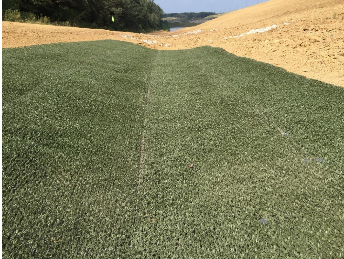
Completed ShearForce10 Installation looking down channel grade
