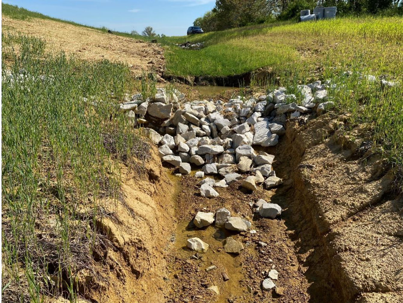
May 1, downstream rock check dam damage
