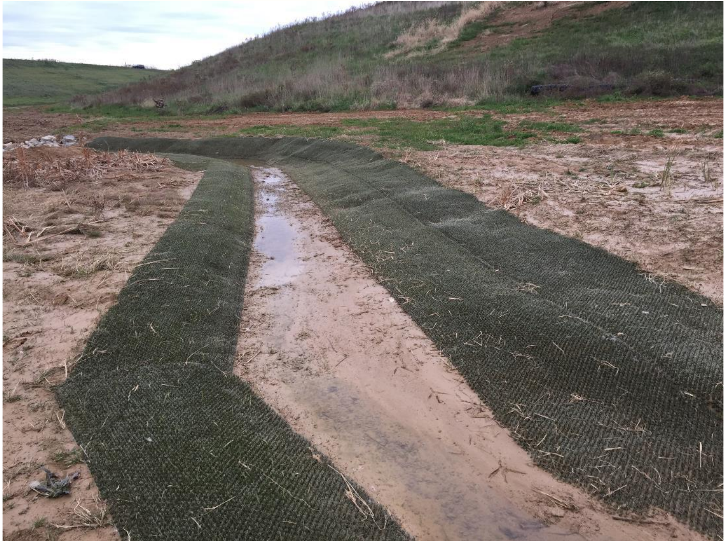
InstaTurf ShearForce10 ECTRM Installed October 25 on seeded streambank
